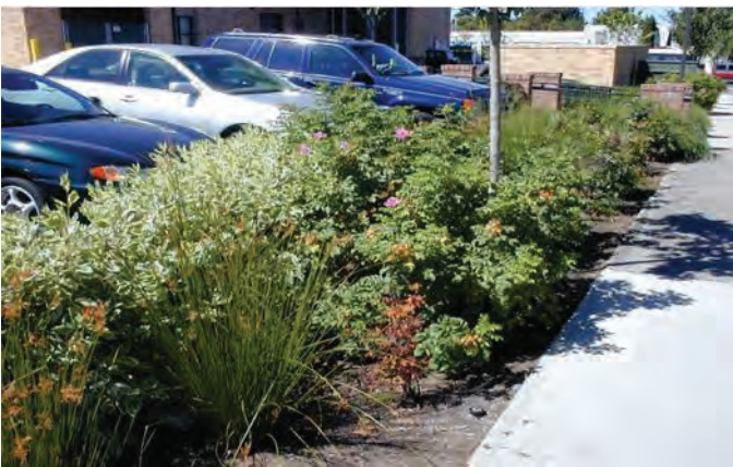
Figure 9. Vegetated Filter Strip (New Seasons 33rd Ave.)
