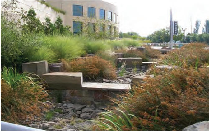
Figure 8. Rain Garden (Oregon Convention Center)
