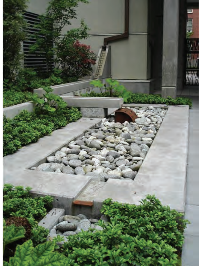
Figure 10. Stormwater Planters (Pearl District)
